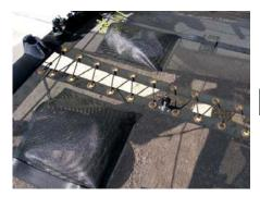
Tie the center lacing line. Start with a bowline knot. Lace the line back and forth taking up slack as you go. When lacing go through the grommets over/under.
